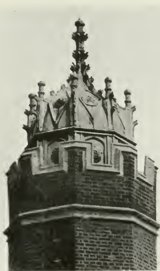
110. Lead Cupola, Hampton Court.
